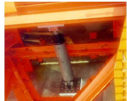
Fig4.2 A 1,000 kN MHD at the Seyhan River Bridge, Adana, Turkey
