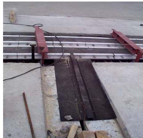
Fig.1.5B A conventional longitudinal joint connected to a DB mat (Humbolthafen Berlin, Germany)
