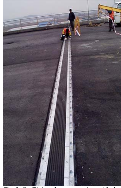
Fig.1.4b: Fixing the mat section with the aluminium clamping section on top of what can be seen left
