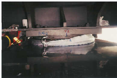
Figure 2: Effects of creep in a PTFE sliding bearing
