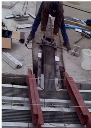
Fig.1.5A: Humbolthafen Berlin, Germany: Vulcanised T-piece that is being prepared to receive another vulcanised butt joint connection on site with a longitudinal DB joint.
