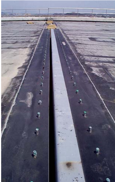
Fig.1.4a: Above: Alternative installation method, example Korean High Speed Railway: Applying the sealing foil and connecting the sealing foil with the adjacent waterproofing layer of the bridge deck
